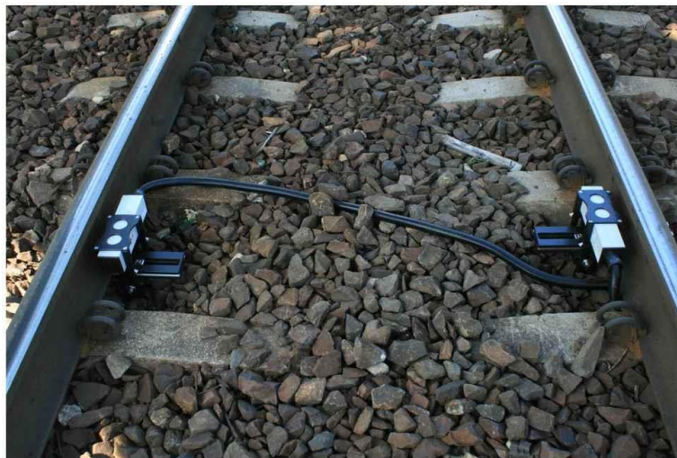
Fig. 2. Two measurement antennas mounted to the rails
