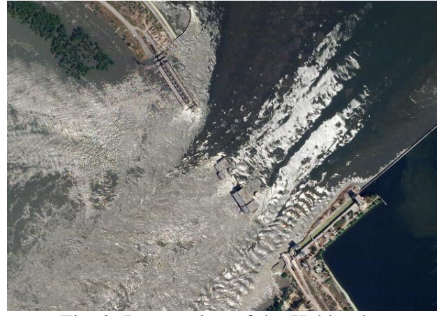
Fig. 2. Destruction of the Kakhovka hydroelectric dam (June 6, 2023)
